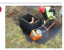
Lay backfill material in 150mm layers, compacting between layers to top edge of chamber
