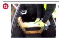
Use bracing if chamber is bigger than 610
